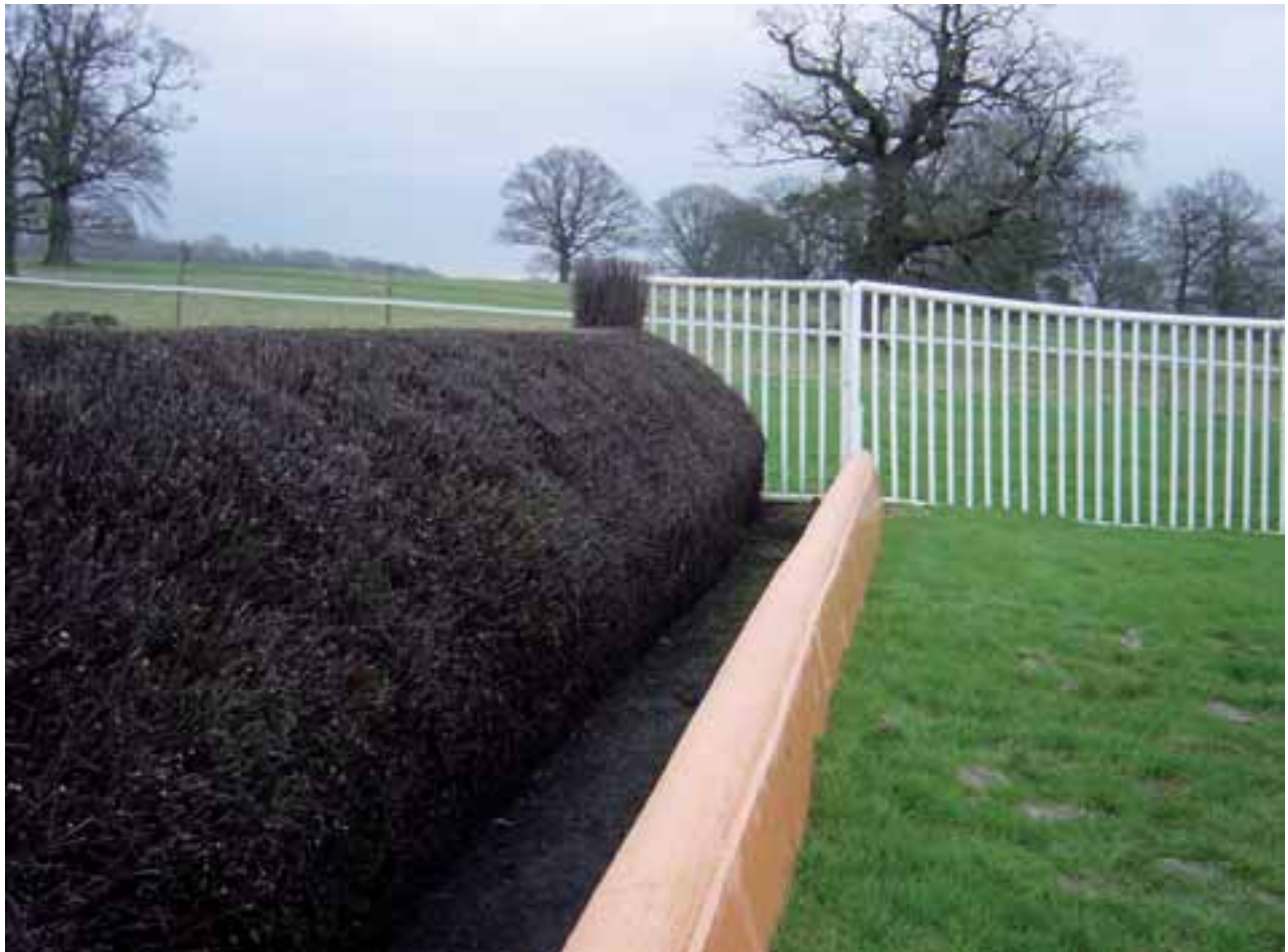
Photo 1.D Open Ditch – Chepstow
