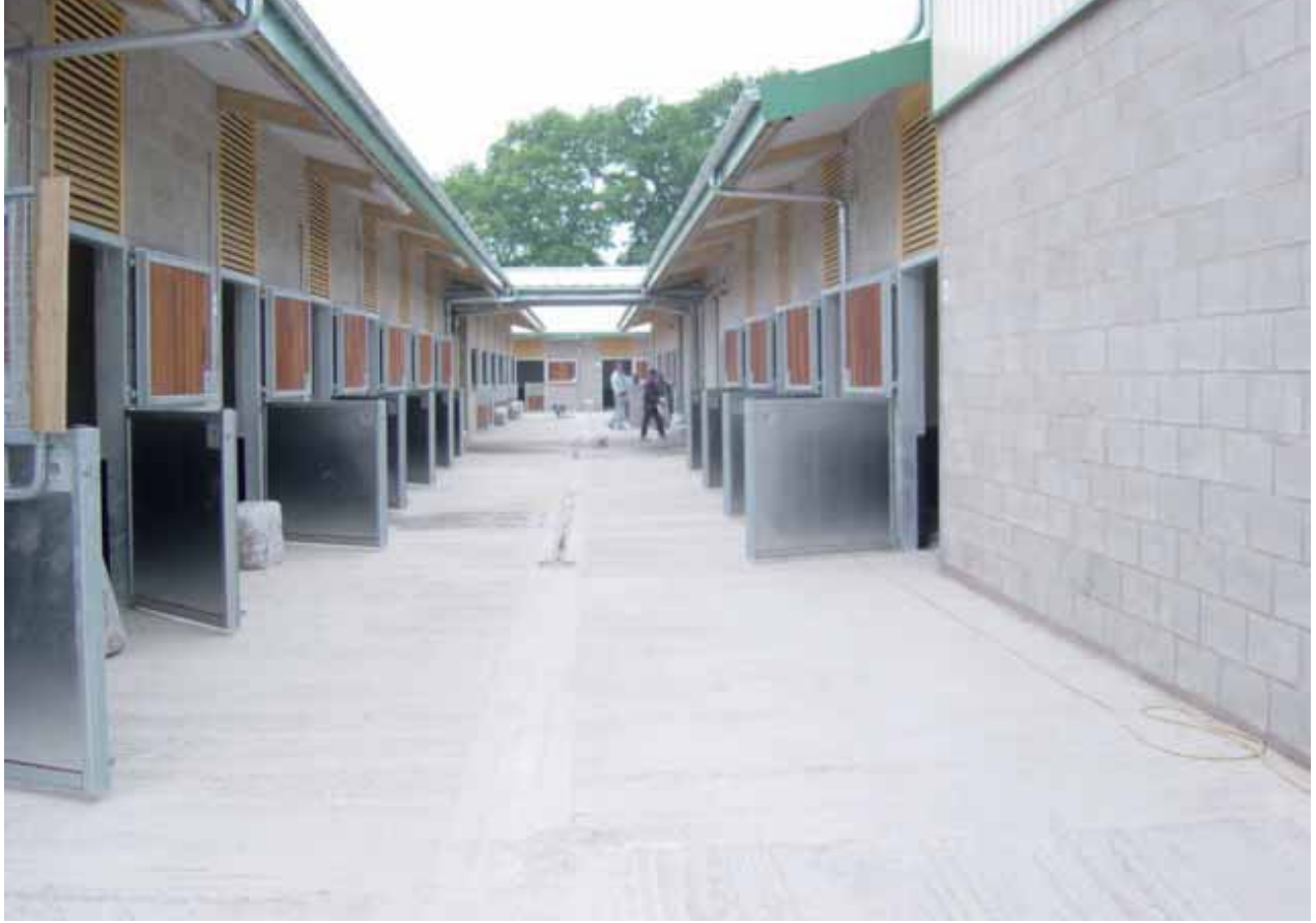
Photo 3.A Official Stables Complex – Warwick
